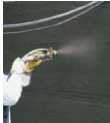
Application Area – Wall Guniting
