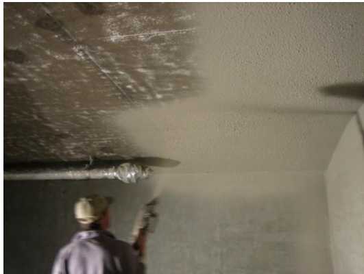
Application Area – Overhead Guniting
